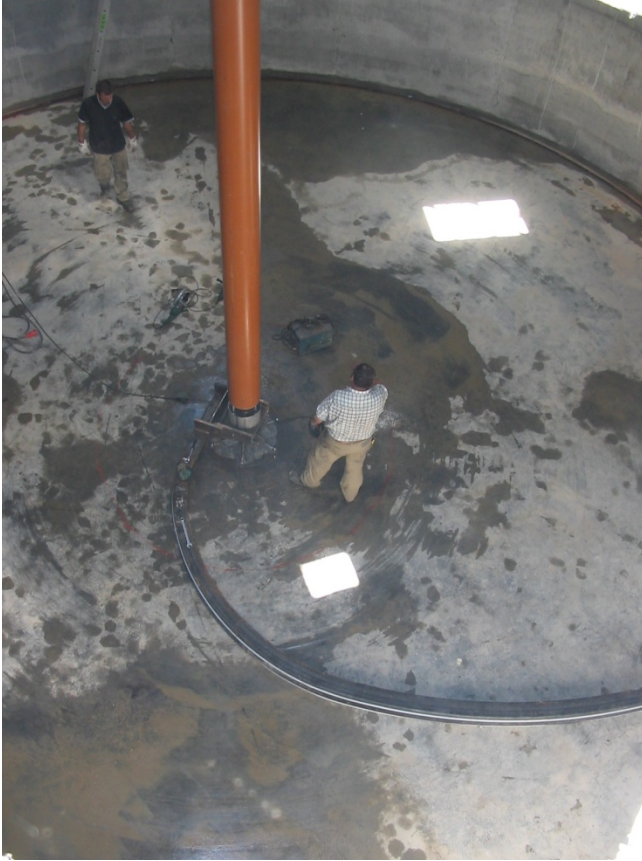
Digester Tank: Floor Scraper
